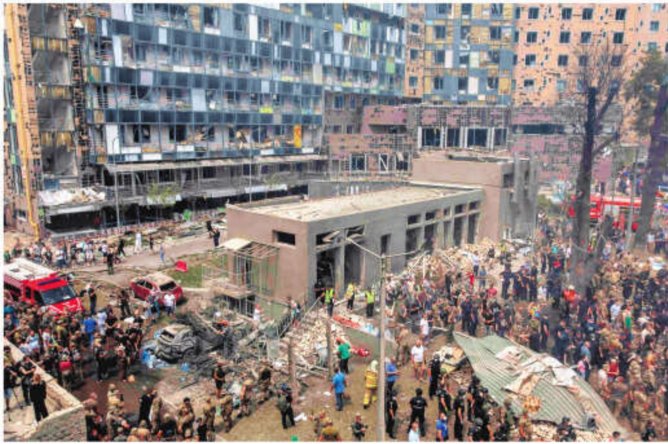
Emergency and rescue personnel along with medics and others clear the rubble of the destroyed building of Ohmmdyt Children's Hospital following a Russian attack in Kyiv on Monday | AFP
